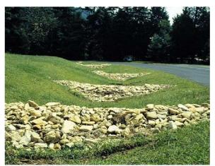
Figure 3: Vegetated swale with check dams (DCR 1999b)
