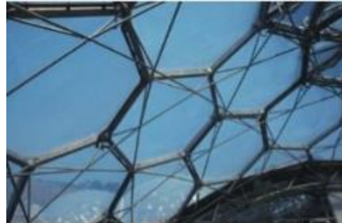
Gambar 6. Rusuk radial dan circumferential tubes
