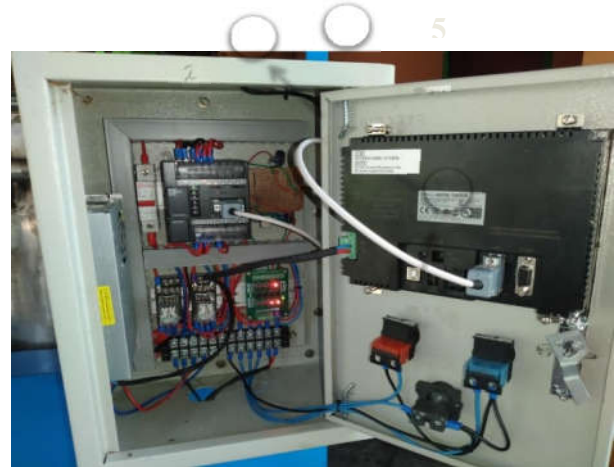
Gambar 13 . Tampilan isi box panel kontrol
