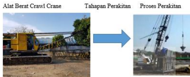
Gambar 6. Perakitan Pipa Tremie
