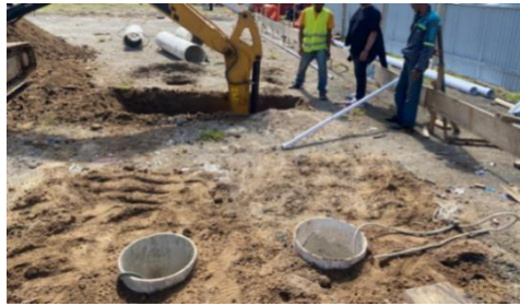
Gambar 3.7 Pemasangan Pipa Casing Bored Pile
