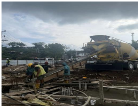
Gambar 3.14 Pengecoran Pondasi Bored Pile
