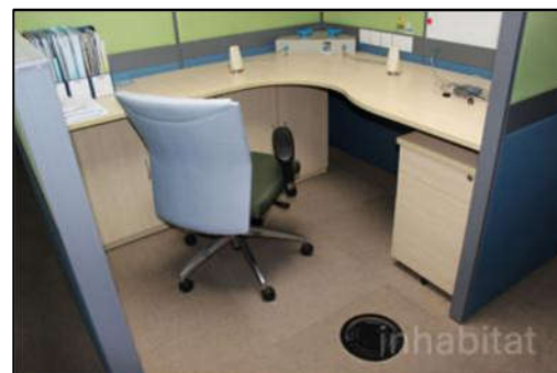
Gambar 13 Lantai Diffusers Sumber : www.inhabitat.com
