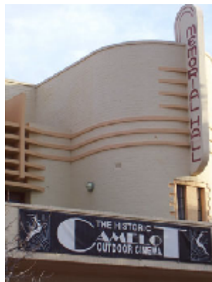
Mosman Park Memorial Hall Architect:Kreitmeyer & Rowe (1939)
