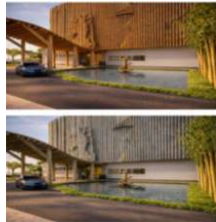
Figure 11. Building Envelope (ulin wood) Before and After weathered
