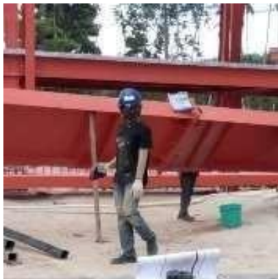
Gambar 7. Proses rafter dilangsir
