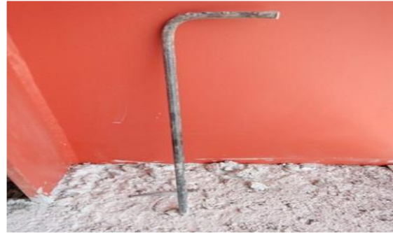
Gambar 7. Tulangan shear connector
