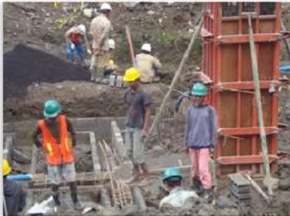
Gambar 3. Bekisting Kolom
