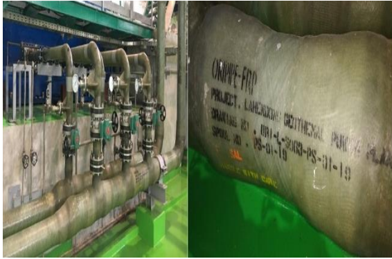
Gambar 11. Generator Air Cooler PLTP Unit 5&6
