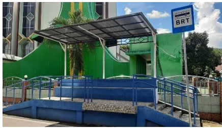
Gambar 11. Shelter BRT Sumber : Survey Lapangan, 2021
