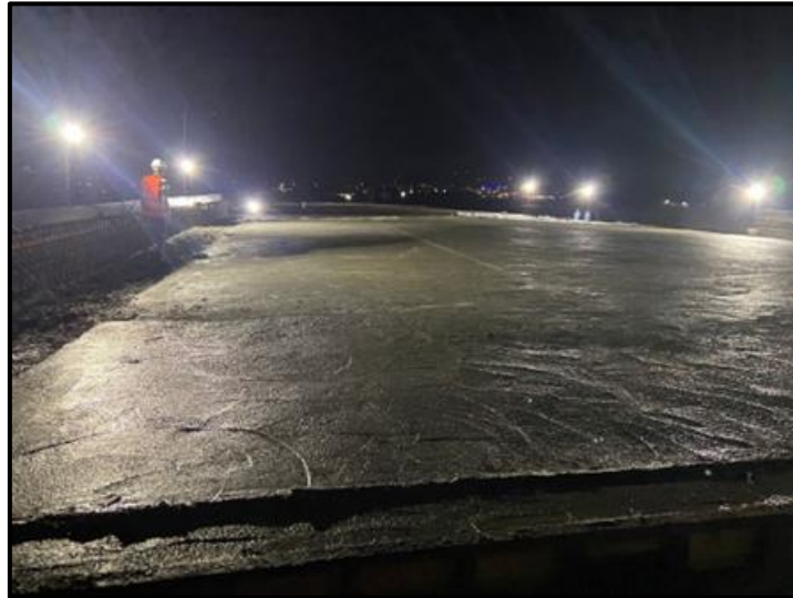
Gambar 20. Finishing Plat Lantai
