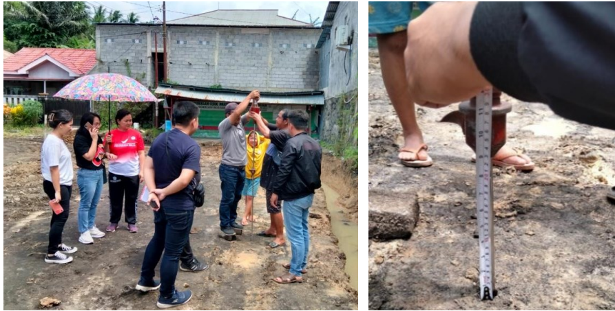
Gambar 4. Pengujian Dynamic Cone Penetrometer
