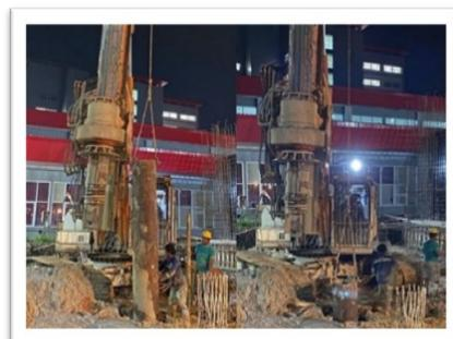
Gambar 8. Pemasangan *Temporary Casing*
