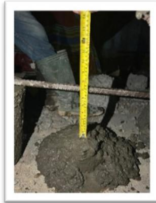
**Gambar 13.** Slump Test
