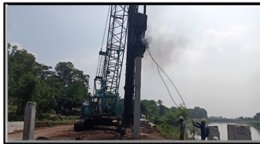
Gambar 22. Pengoperasian Diesel Hammer
