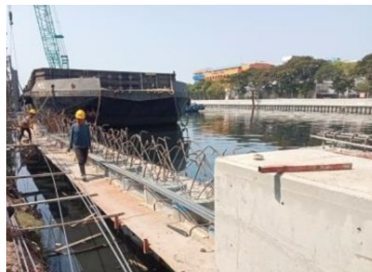
Gambar 8. Pekerjaan Beton Pengisi Grouting Connector
