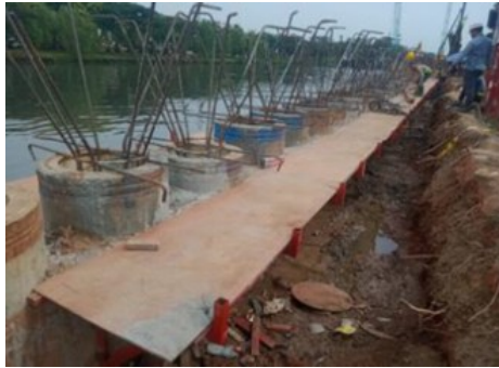
Gambar 9. Platform Bekisting
