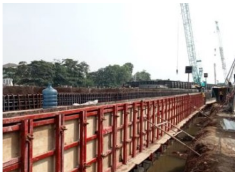
Gambar 10. Bekisting Multipleks 18 mm
