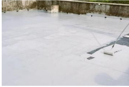
Gambar 10. Screed Atap Dak
