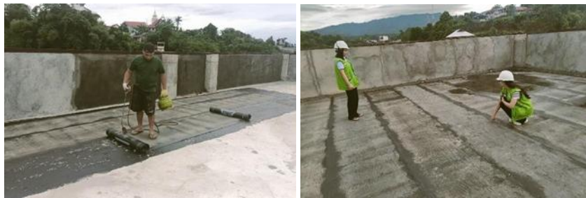
Gambar 11. Waterproofing Atap Dak
